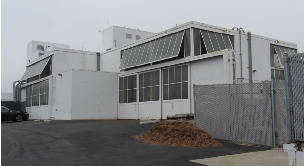
Figure 3 -View of Central Plant
