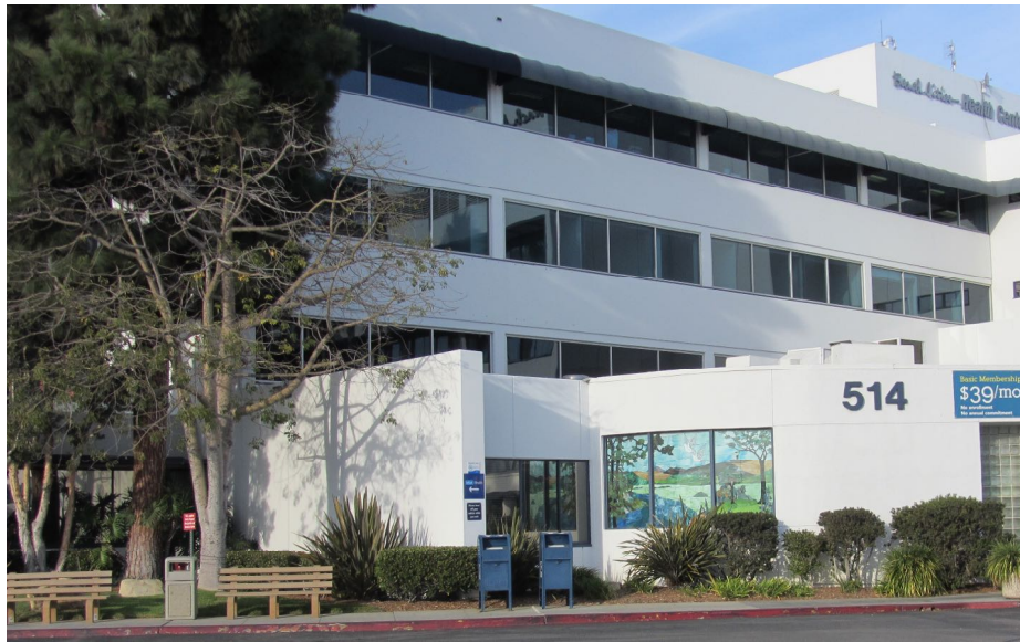
Figure 2 - View of South Side of North Tower
